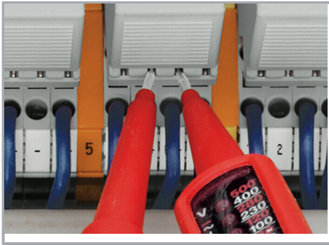
Function testing via touch-proof test slots
