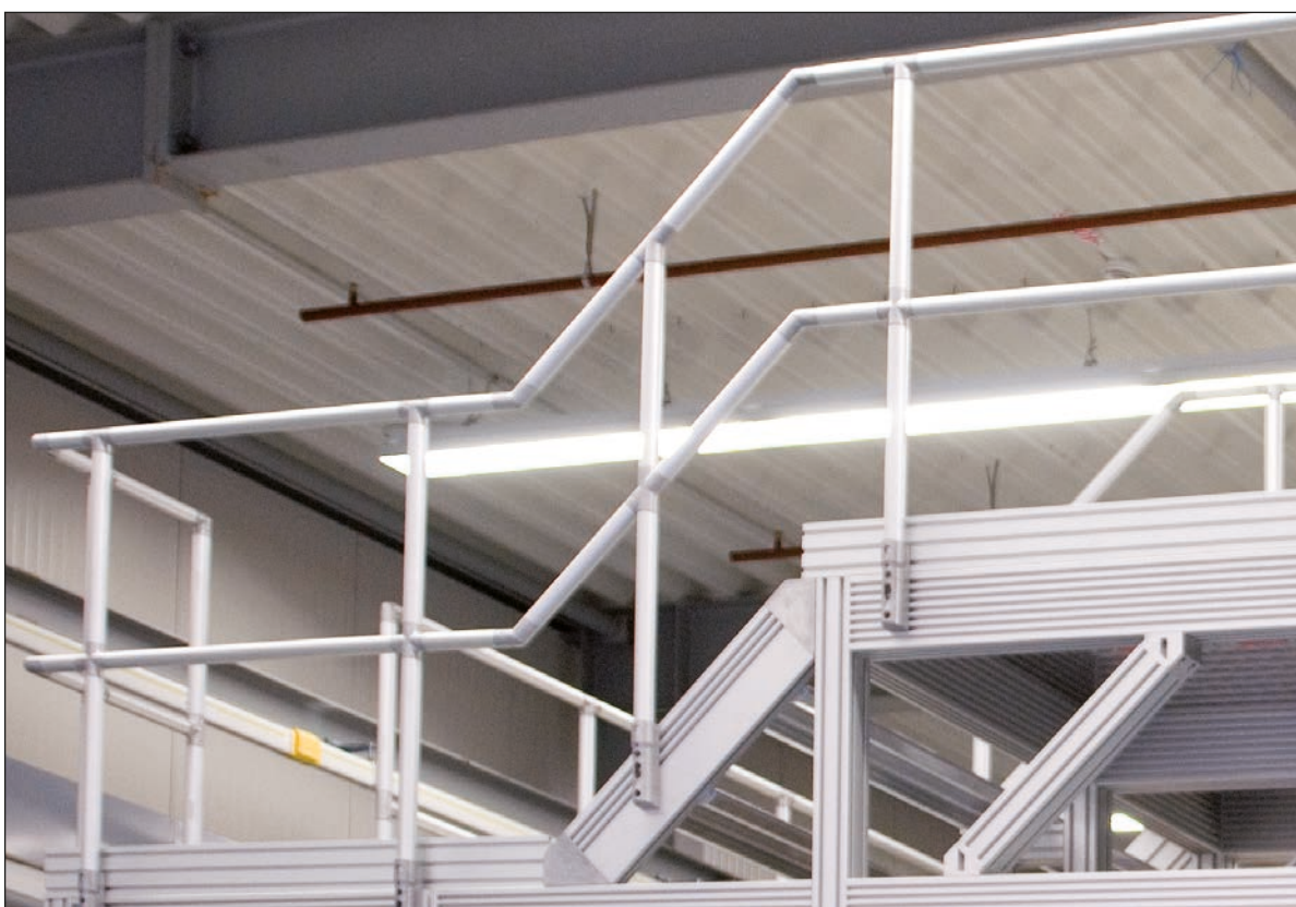
Staircase between two operating platforms.
