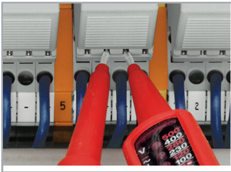
Function testing via touch-proof test slots
