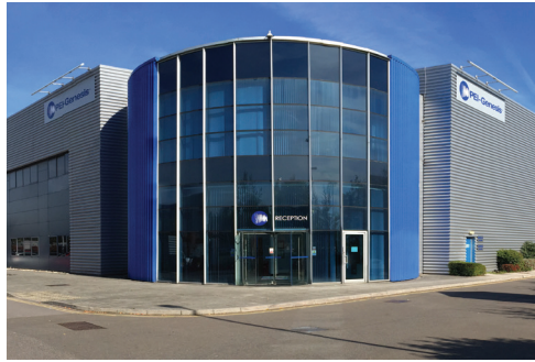
European Headquarters & Production Facility, Southampton, UK
